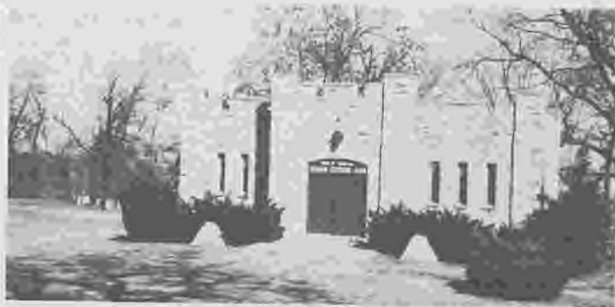
Fort D, 1861 - largest of four forts built in Cape Girardeau
